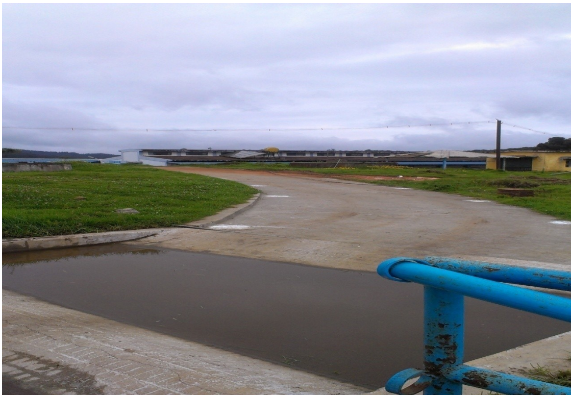
Tyre Dip at Entry
