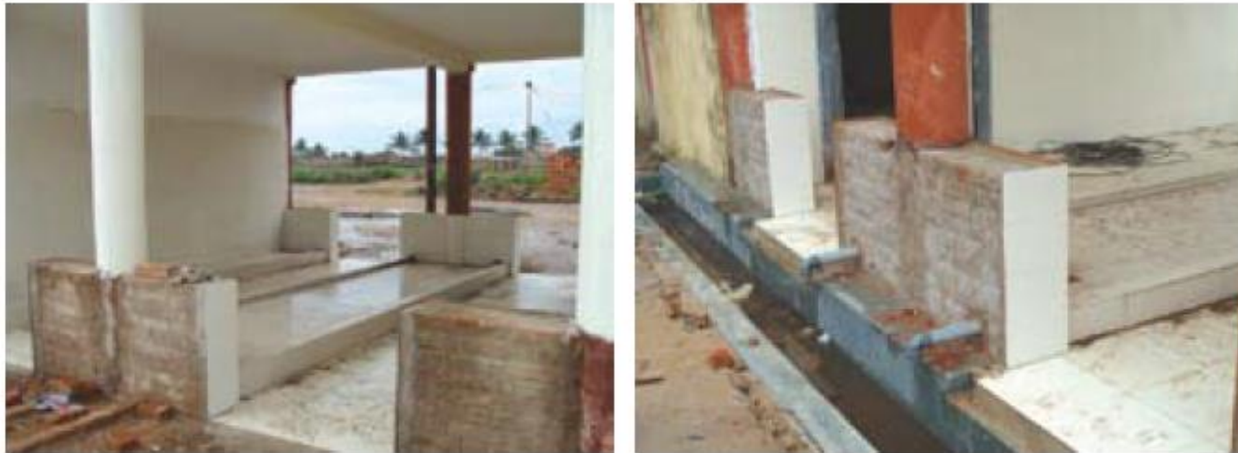
FIGURE 31 Crouching-only sorting platforms under construction
