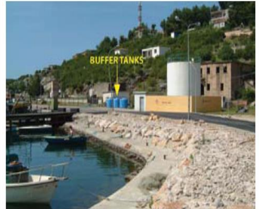
FIGURE 1 Buffer tanks to even out fluctuations in town mains supply
