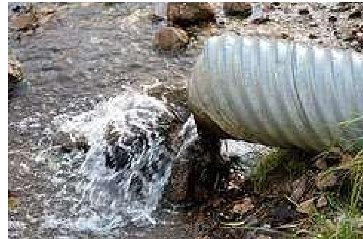
Fig.3 (a and b) Industrial waste water polluting water bodies.
