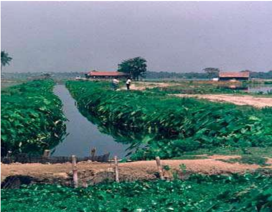
Fig. 13 (b) Open channel through which sewage is flown to the pond.
