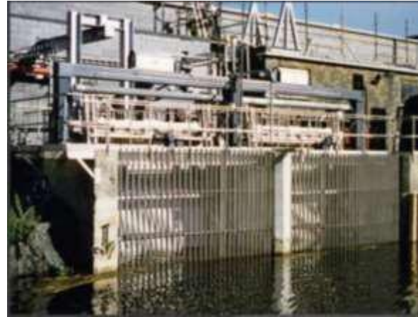
Fig. 6 (b) Fine screener for water plants, leaves etc.
