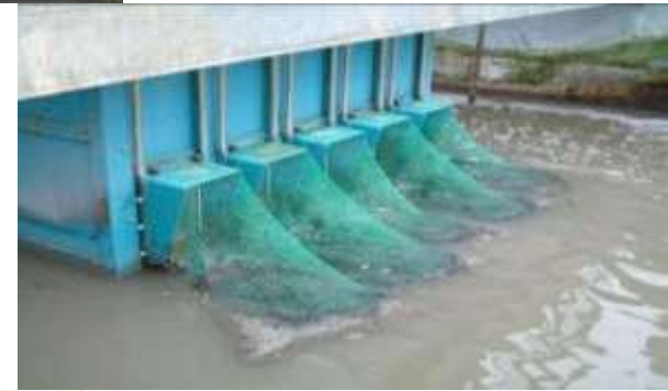
Fig. 6 (b) Fine screener for water plants, leaves etc.
