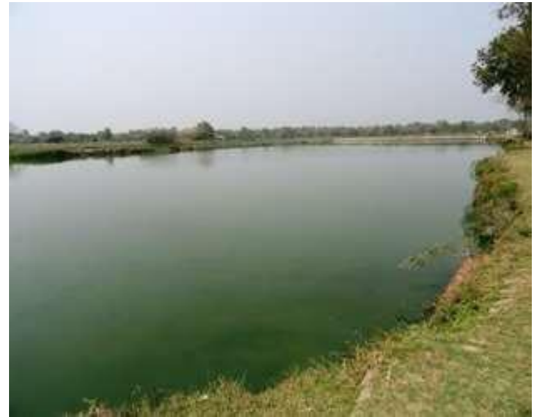
Fig. 11(a) Oxidation pond.
