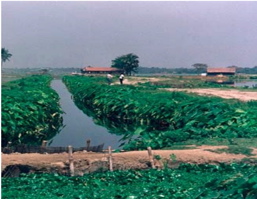
Open channel through which sewage is flown to the pond.
